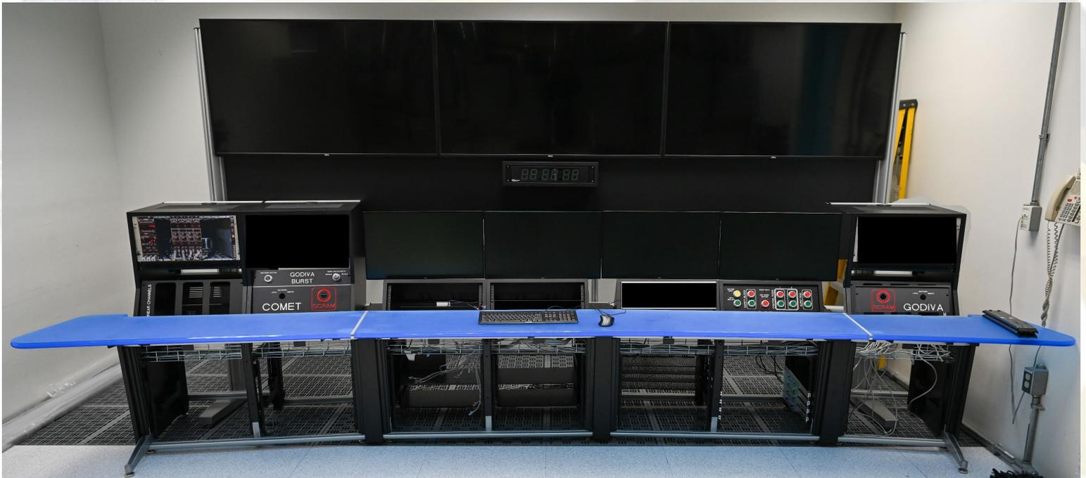
▲ Upgraded control console with larger monitors installed in Control Room 2.
